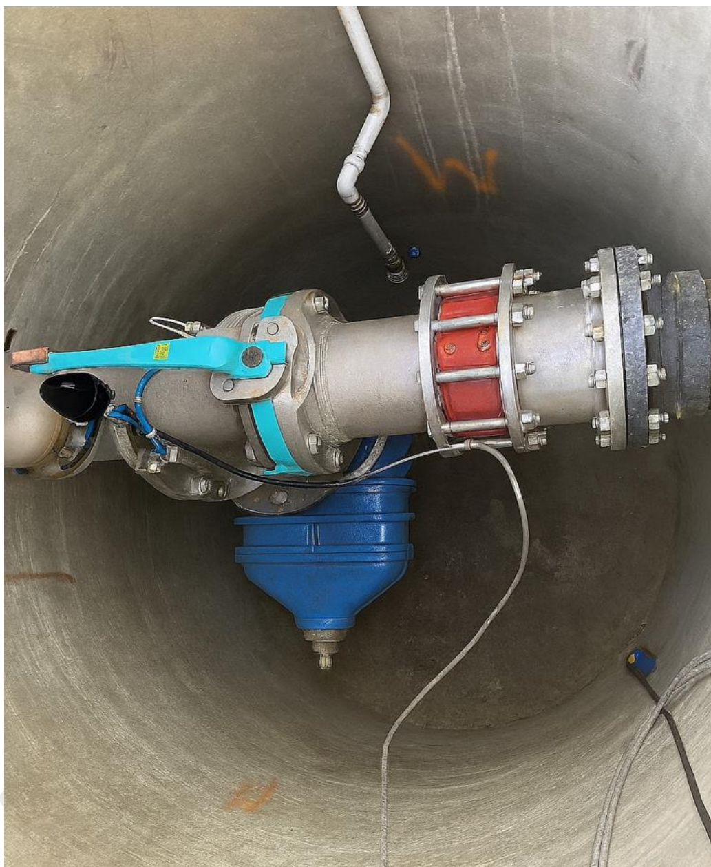
Figure 11 – Below-ground installation of headworks
