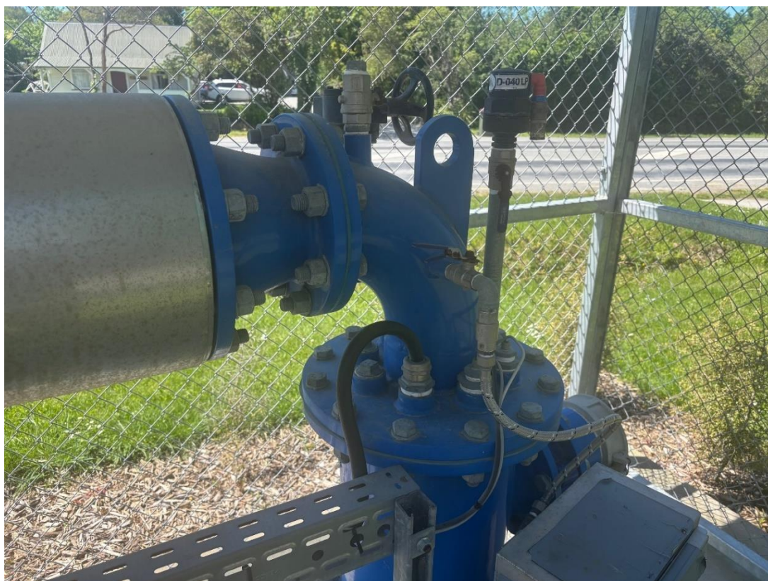
Figure 17 – Drinking water supply bore head componentry
