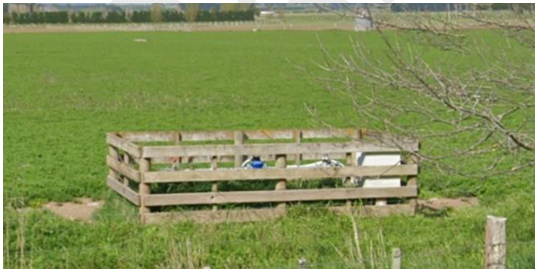
Figure 18 –Agricultural water supply bore head
