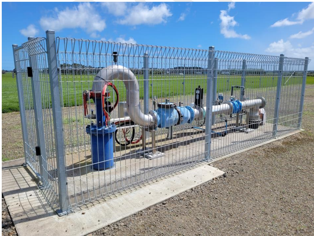
Figure 16 – Drinking water supply bore head (variation)
