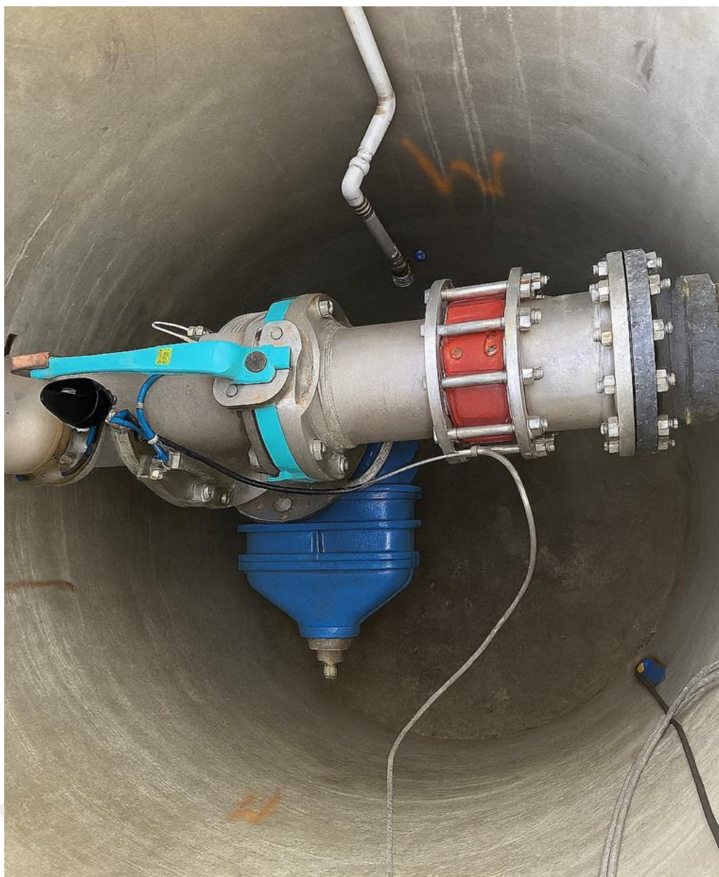
Figure 11 – Below-ground installation of headworks
